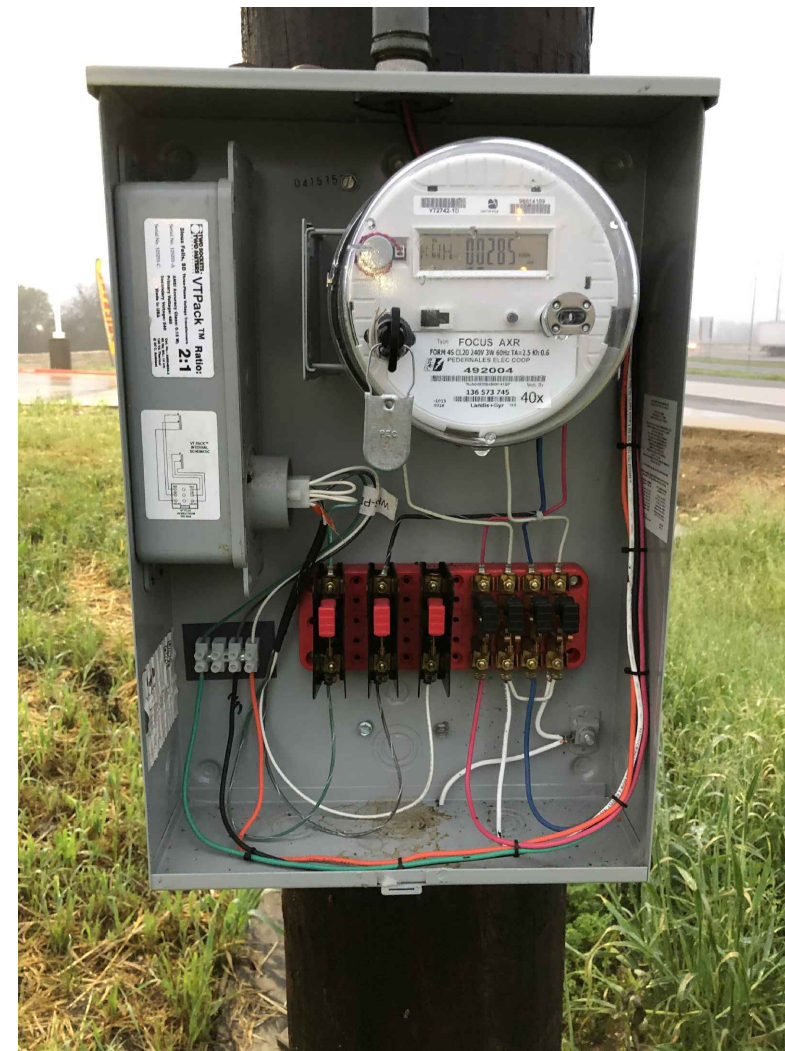
METER INSTALLED
